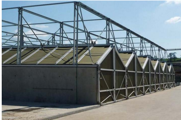
Figure 1.4 – An example of a covered clamps composting system (covered with metal sheets)
