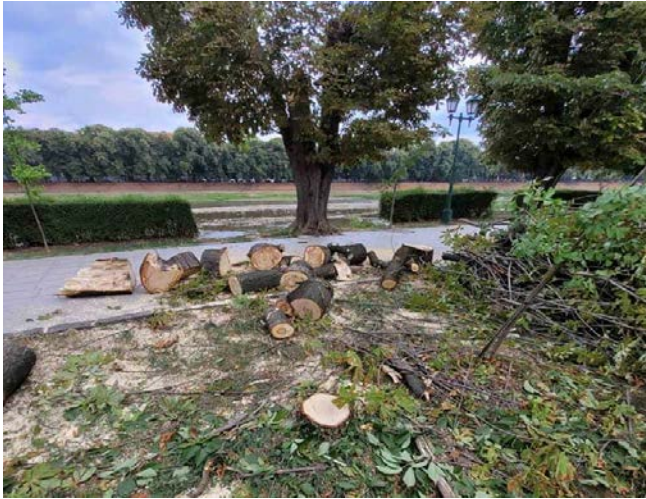
Trimming and removal of trees
