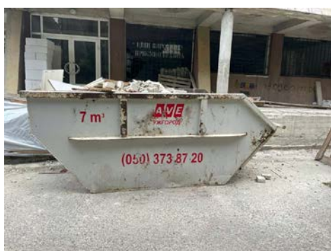
Container for collecting CDW
